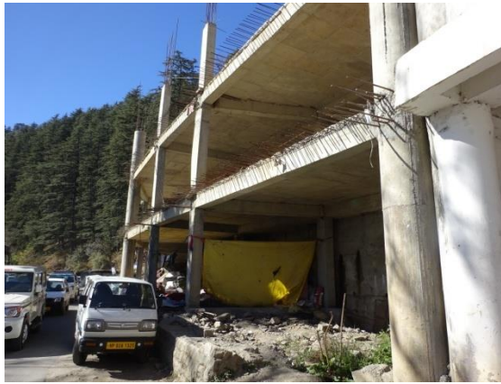
Figure 5.1 Car parking cum-shopping complex at Sanjauli
